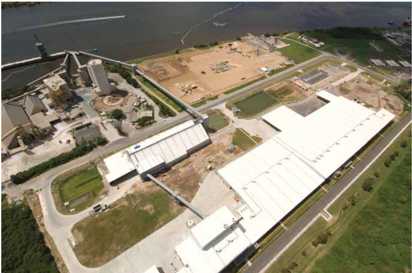
Boral Plasterboard plant at Pinkenba, Queensland, uses recycled water in the manufacturing process to reduce the dependence on public water resources.
